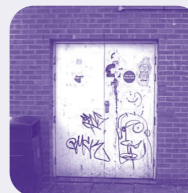
▲ Fire exit before
