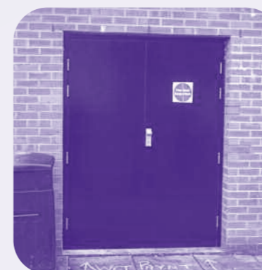
▲ Fire exit after
